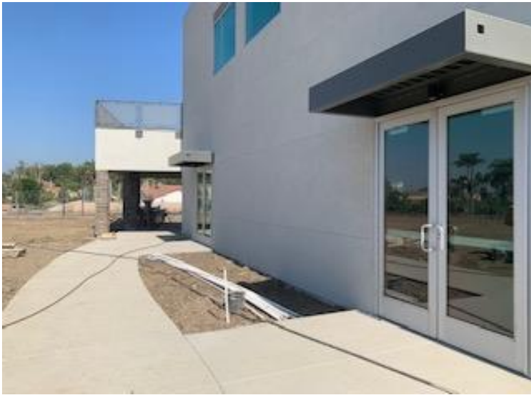
Side entrance to main meeting room
