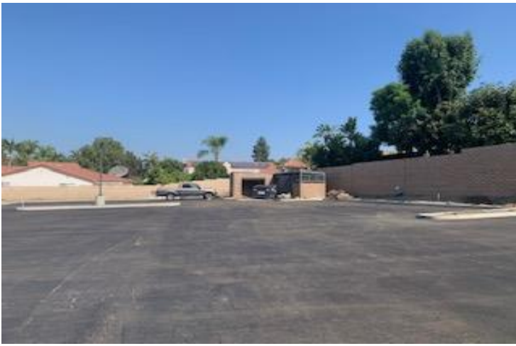
View of maintenance building/trash receptacles
