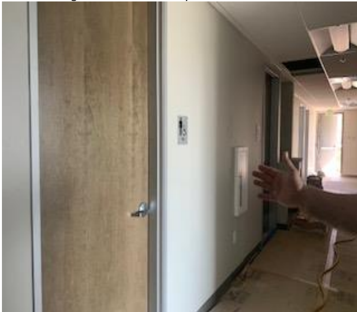
A view down the hall at the bathroom and classrooms upstairs
