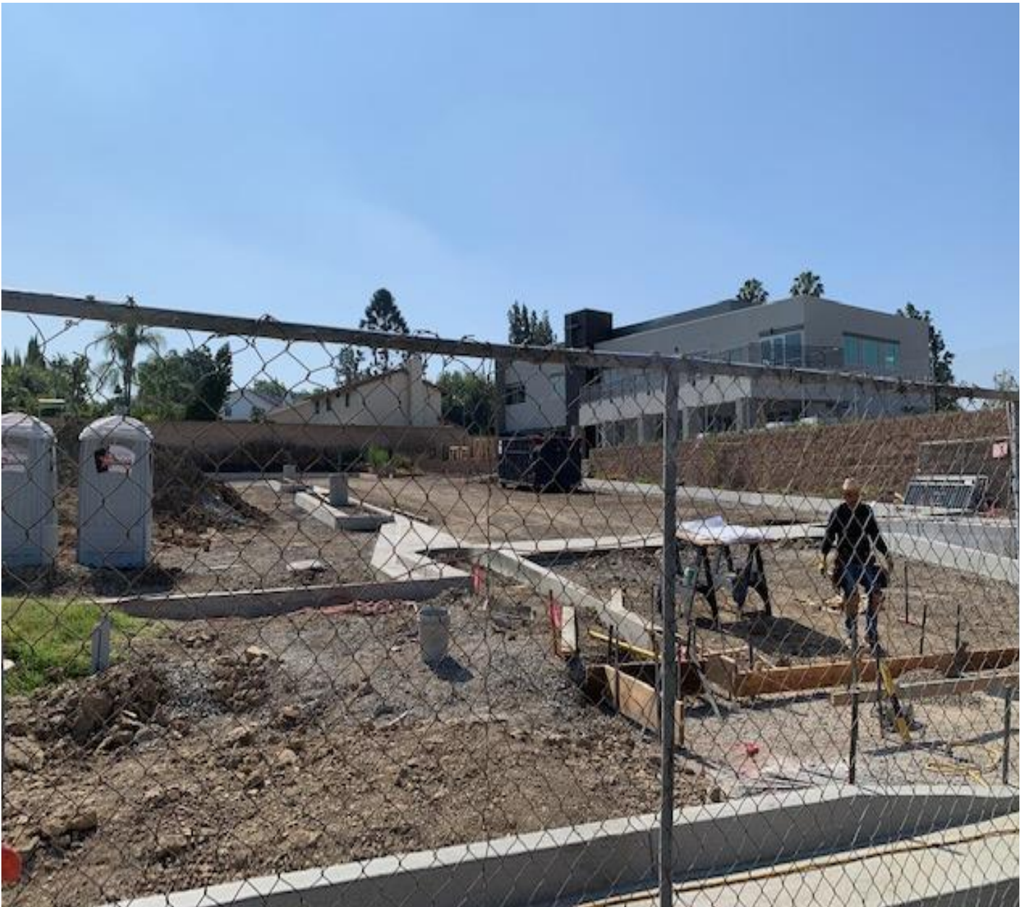
Still working on the framing of the parking stalls, driveway, and curbs .....
