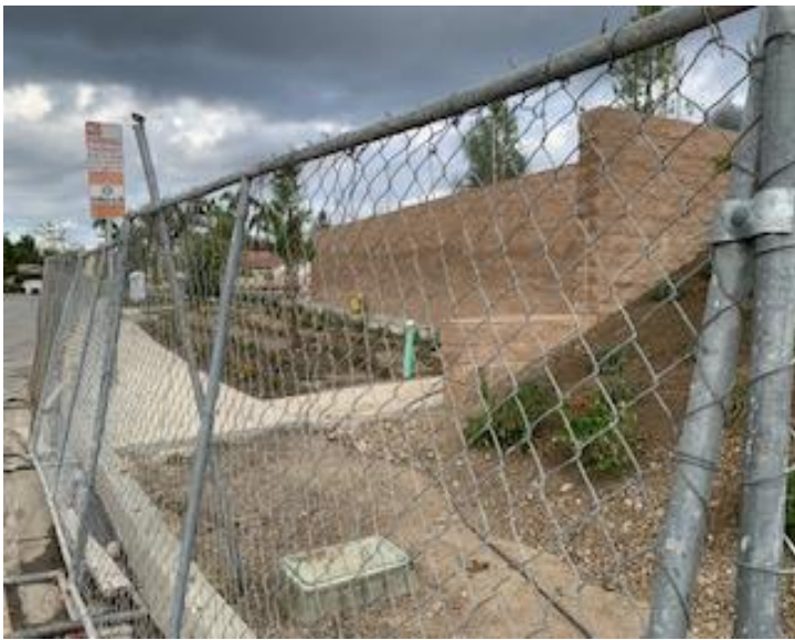
Sidewalk to be completed on Sterns
