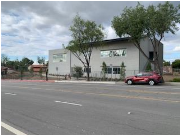
View from across the street on Foster
