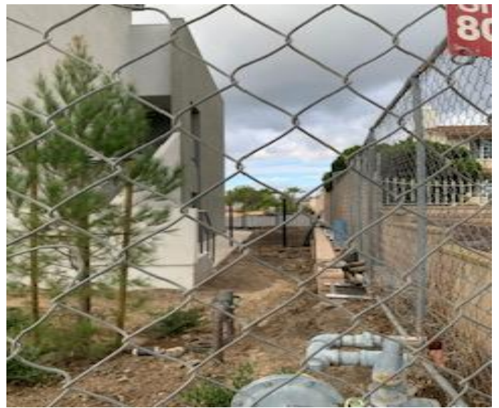
Fence and gates still to be completed
