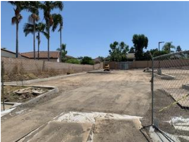
Back fence installed!
