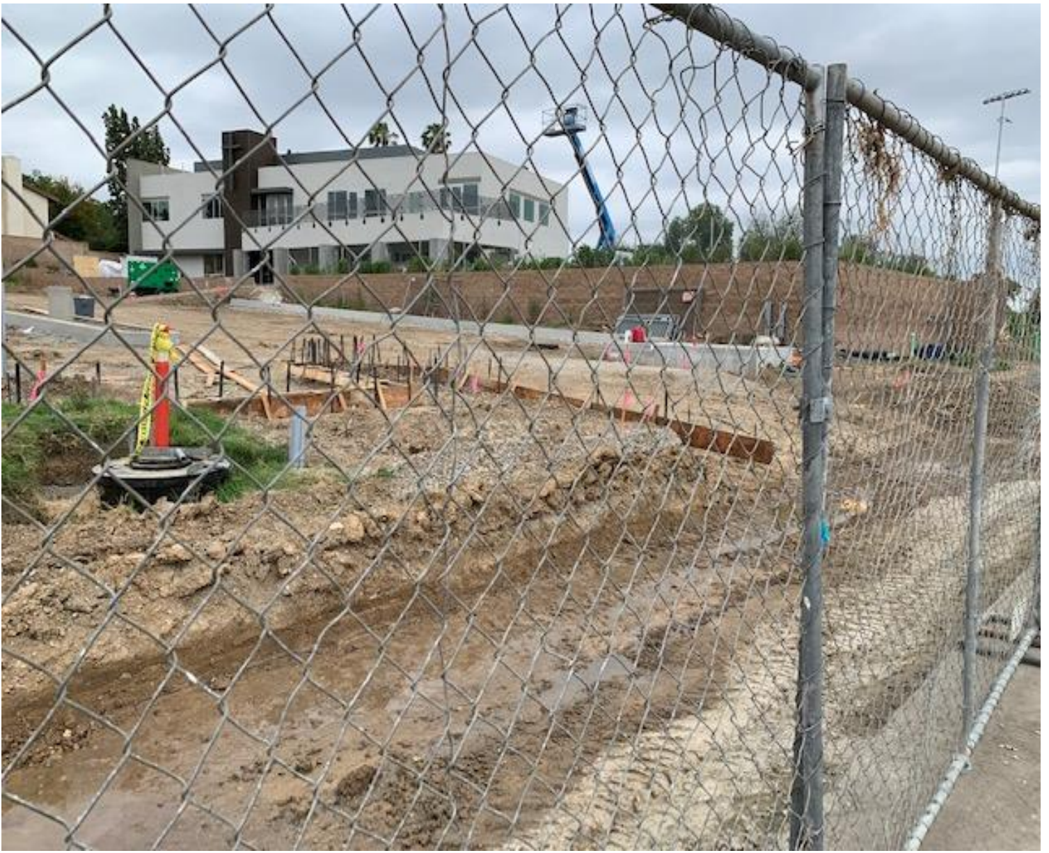
Forms are going up for curbs and driveways. Slow but sure.....
